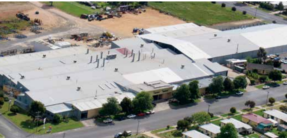
All steel and assemblies are kept under cover.
